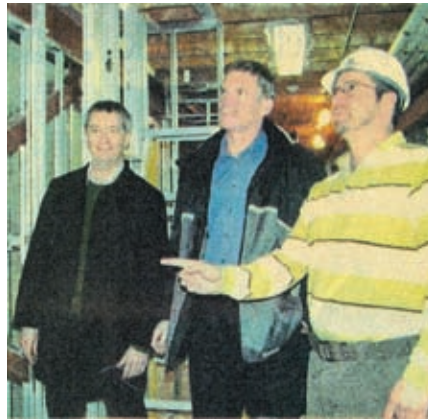
Dr. Tom Crichton (left), David Courtemanche and Frank Taylor check on the progress of the Pioneer Manor site of the City of Lakes Family Health Team. Pioneer Manor is one of four sites for the team, and it should be renovated by June. The other sites will be in Val Caron, Chelmsford and Walden.
